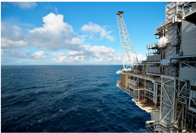
Figure 1: Tendeka has secured the world's largest sand and inflow control contract for the Troll field on the Norwegian continental shelf Photo credit - Harald Petterson, Equinor
