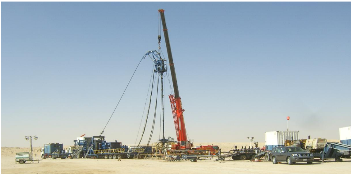
Figure 6 Surface equipment required for the Production Log surveys
